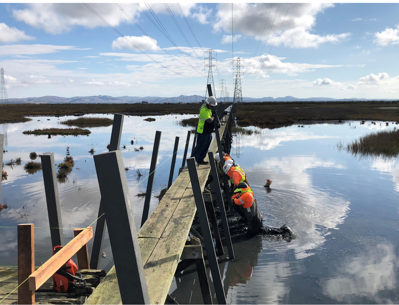
Figure 4. Crew installing boardwalk posts by hand in tidal marsh.
