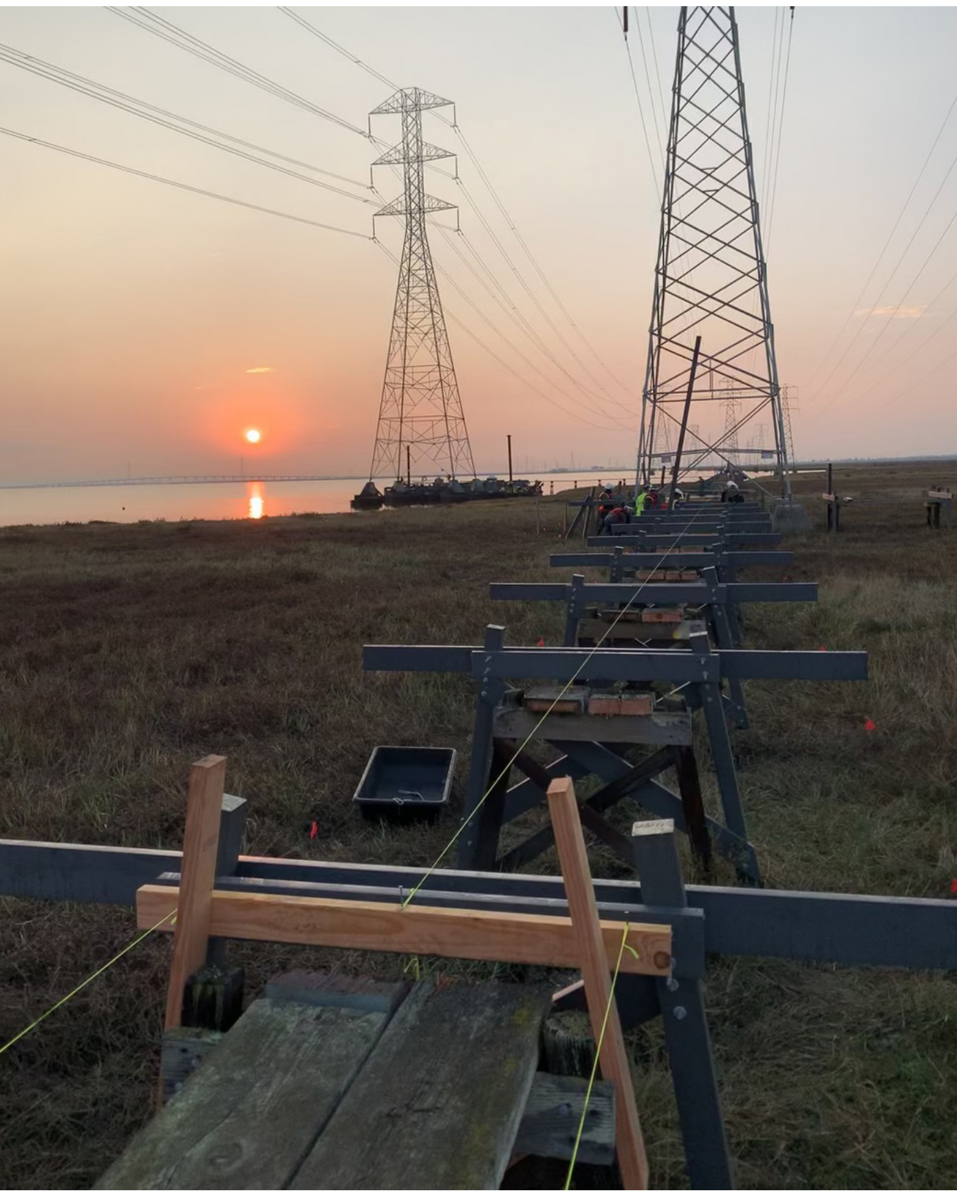
Figure 5. New boardwalk being constructed over an existing boardwalk. Staging barge visible in background.
