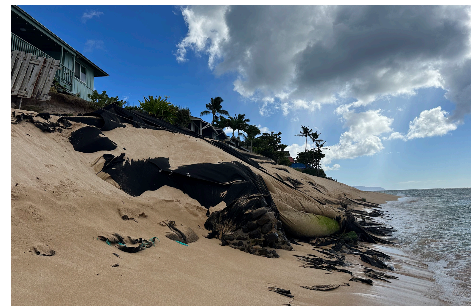
A geotextile sandbag structure has protected private property, but results in a total loss of nesting habitat.
