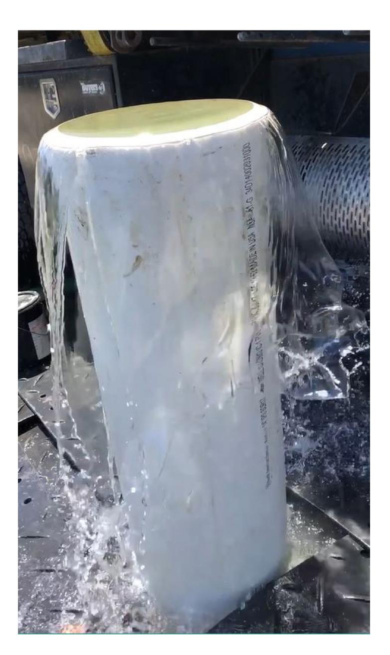
Artesian water flow from PVC casing of new South Bay Well
