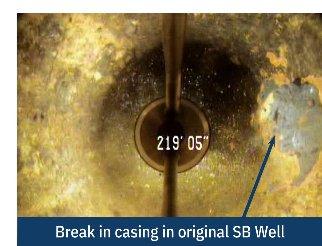
In December 2013, the District hired a well driller to rehabilitate the well. Rehabilitation consisted of installing an 8-in. diameter PVC casing inside the original casing. The bottom of the PVC casing extended to 424 ft bgs (6 ft above the original total depth). Sixty feet of 0.032-inch slot PVC casing was installed at the bottom, above which 180 ft of blank casing was installed to a depth of 184 ft bgs.
